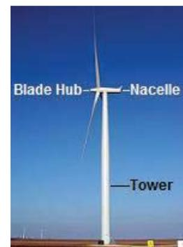
Figure 1. Wind Turbine Components
